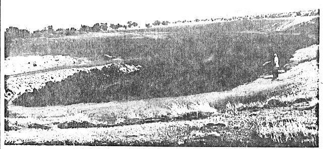
Huge dump ponds will become common sights if coal slurry pipelines are granted eminent domain. During a pipeline rupture or power failure, the slurry must be flushed from the pipe into ponds or on the ground. When the water evaporates, there is the danger of thousands of tons of coal dust blowing across the countryside.
