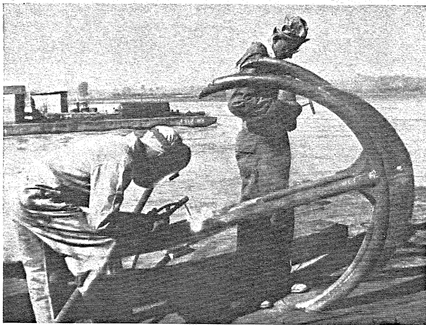
Welders exercise their ingenuity to build up an anchor on one of the crossings of the Missouri river. Photo taken in 1948.
