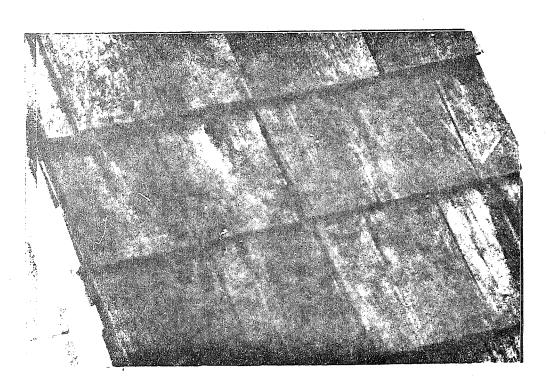
Dark areas on shingles where rockets were fired are discolored from burned powder. Not burns on shingles.
