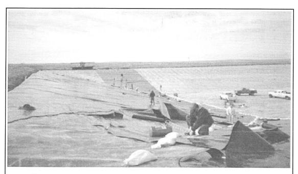
These two pictures depict animal-waste lagoons. The picture above is a lagoon being built for hog wastes in southwest Kansas. A plastic liner is being installed on top of the compacted clay liner, although this is not the norm. The trucks are parked in the bottom of the lagoon, which gives a sense of its size.
