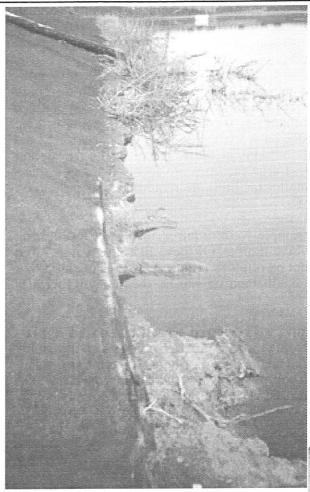
These pictures depict some potential problems with animal-waste lagoons. The lagoon on the left shows signs of erosion where the clay liner has been partially washed away. The operators have installed a fabric to help control the erosion, but it clearly hasn't eliminated the problem. One possible impact is that the liquid will seep out of the lagoon at a faster rate than it should.
