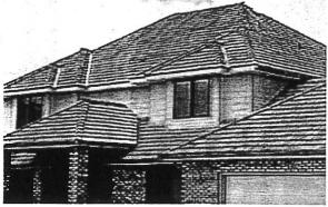
Taper-sawn shakes are as thick as hand-split shakes and are sawn smooth on both sides. They come in three grades: Premium and Grades 1 and 2.
