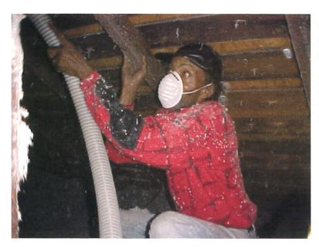
This worker is installing attic insulation in a kneewall section of the attic.
