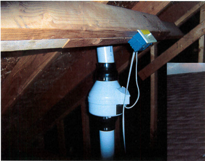
Attic installed radon fan
