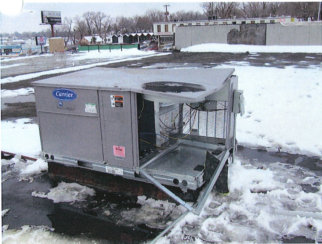
New Air Conditioner Unit stripped on rooftop.
