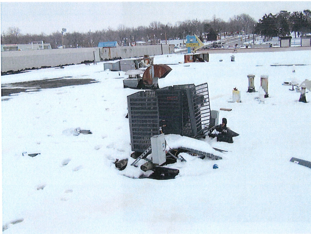
Multiple Air Conditioner Units stripped.
