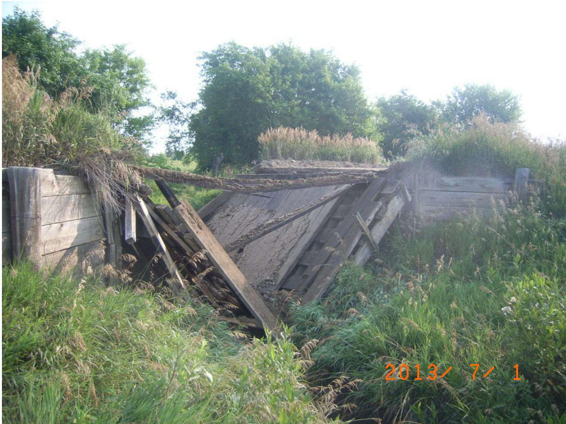
Figure 6 Another timber bridge collapse due to overweight
