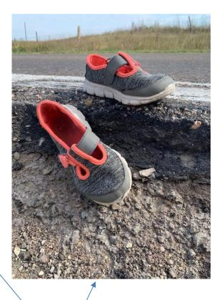
Photos showing deterioration of the white line on Hwy 156; one with Mary Jo's shoes.
